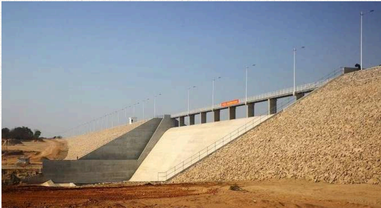
Downstream face of Mwomboshi dam and spillway
