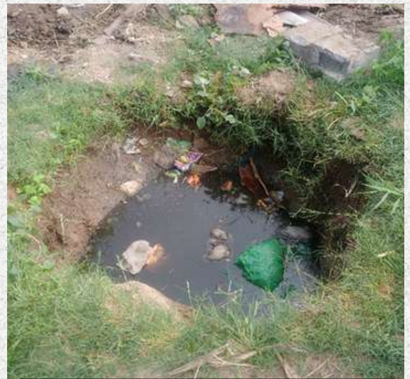
Effluent at the inspection chamber
